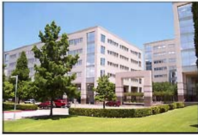
IBM BLDG 904 SOLUTIONS EXPERIENCE LAB
