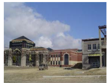
STEVENS HIGH SCHOOL UNDER CONSTRUCTION
